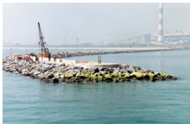
Figure 5: Breakwater constructed in New Ennore coal project
