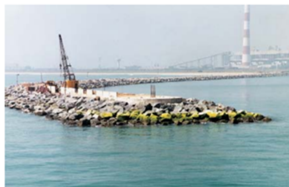
Figure 5. Breakwater constructed in New Ennore coal project ( http://www.ennoreport.gov.in/ )
