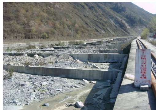
Photo 7 The downstream, drainage channel
